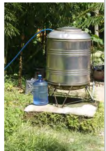
The stainless steel tank here is a 200 liter tank that is filled by the trickle of water from the cistern up on the side of the hill. Once the new cistern is built, the better flow will fill it much more quickly.
