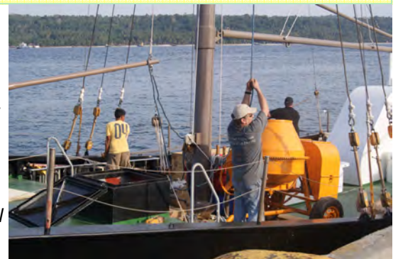
Men aboard RIM Nativa loading cargo and equipment for the voyage to Balut Island. Pastor Britt Dupree of Central Baptist Church, Bastrop, Louisiana hauls on the line as we swing sacks of cement onto the ship.
