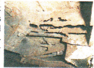
UNDERSIDE CORROSION
