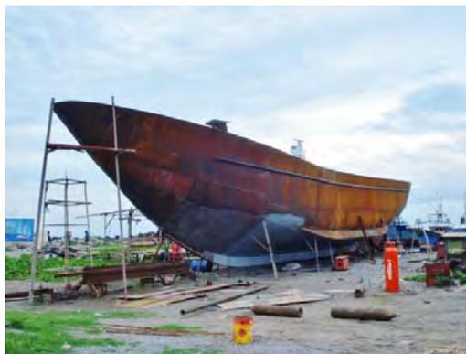
The hull's deep keel is just about finished in all the forward section as can be seen in this photo of the starboard side. This keel is filled with concrete to give her added ballast. Once the work is completed in the after section of the ship, work will begin on the railing, the deck house and wheel house through July and August. Once back in the Philippines in mid-August, I will begin work on the masts, booms and spars, hoping to have that work accomplished by mid-October.
