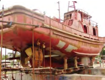
...A large steel tugboat designed and being constructed in the SAFI yard is one of three current projects underway by the company. MSV Nativia II will be laid up adjacent to this vessel.
