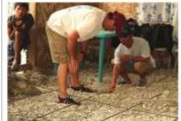
Pastor Nelmar Sumatra setting the reinforcement steel for the floor
