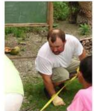
Billy Pearson helping with the lay-out for the floor
