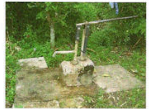
Newly repaired water pump in the church
